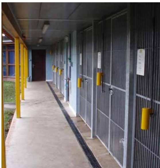
Protected external runs (showing drainage)
